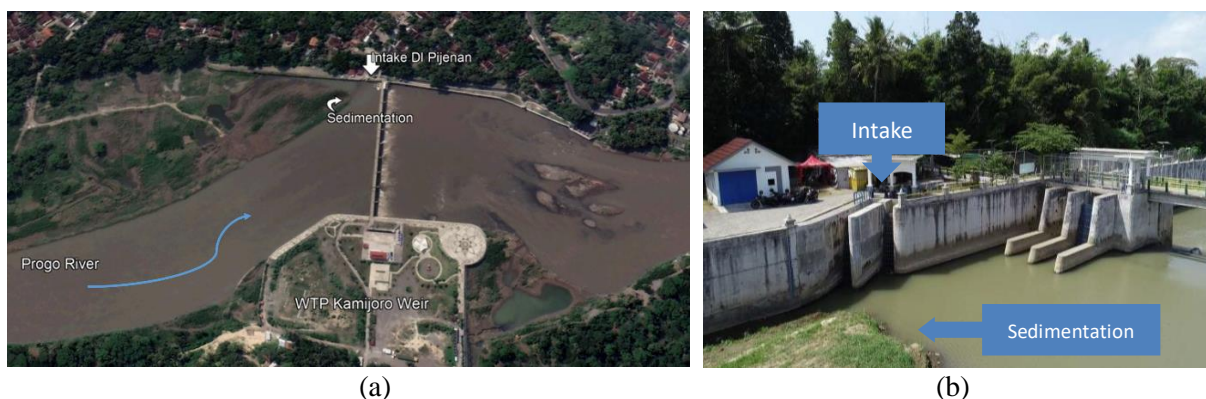
Figure 2 (a) Existing Intake Conditions (b) Sedimentation occurs upstream of the intake
